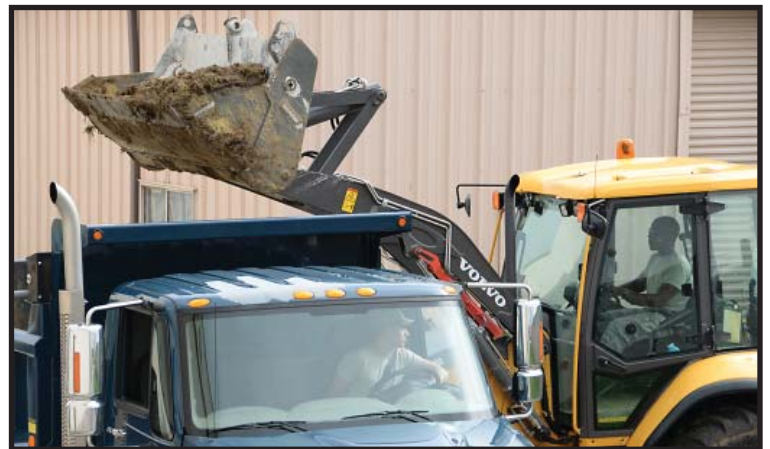
U.S. Air Force Airmen with the 181st Civil Engineering Squadron load piles of dirt from a construction site into a dump truck at Hulman Field, July 12, 2015. (U.S. Air National Guard photo by Airman 1st Class Kevin D. Schulze)
