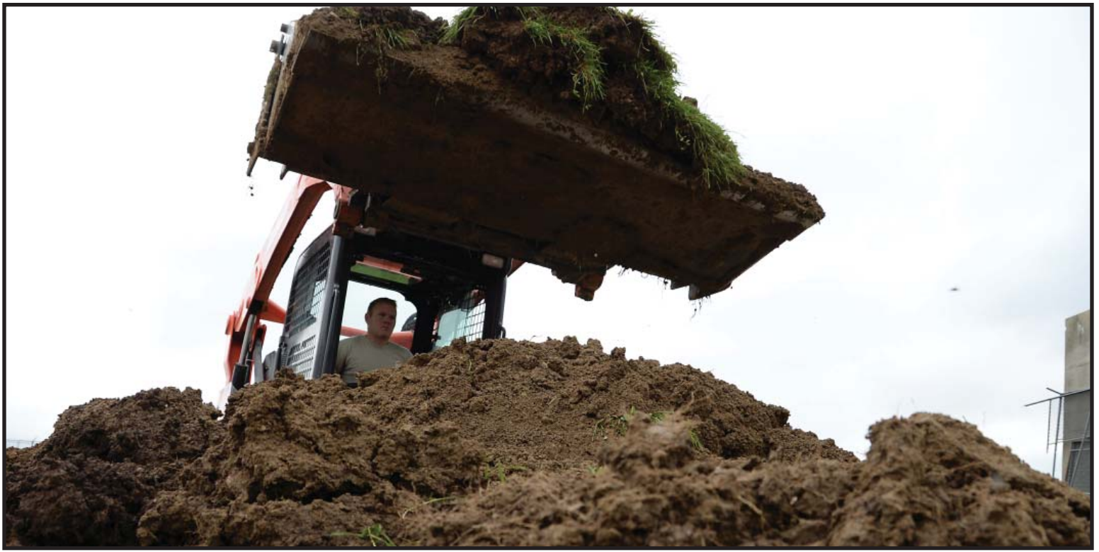
U.S. Air Force Airman with the 181st Civil Engineering Squadron clears dirt from a construction site at Hulman Field, July 12, 2015. (U.S. Air National Guard photo by Airman 1st Class Kevin D. Schulze)
