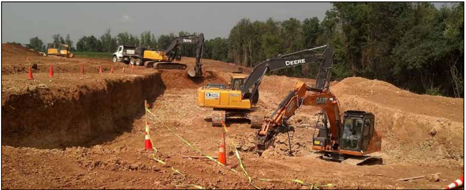
Heavy equipment operators from the Prime BEEF units at Hulman Field, Pittsburgh, and St. Paul excavated 42,000 cubic yards of soil and rock to construct a retention pond and drainage ditches. This is the first phase of the construction of a 110 acre sports and recreation complex for the town of Chippewa Falls, Pa.
