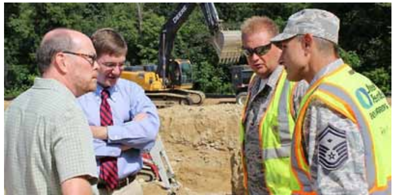
Airman from the 181st CES and 131st CES, St Paul, MN, enlarge a drainage structure opening to accept a larger drainage pipe. The structure was used in the drainage system at the Chippewa Falls sports and recreation complex.
