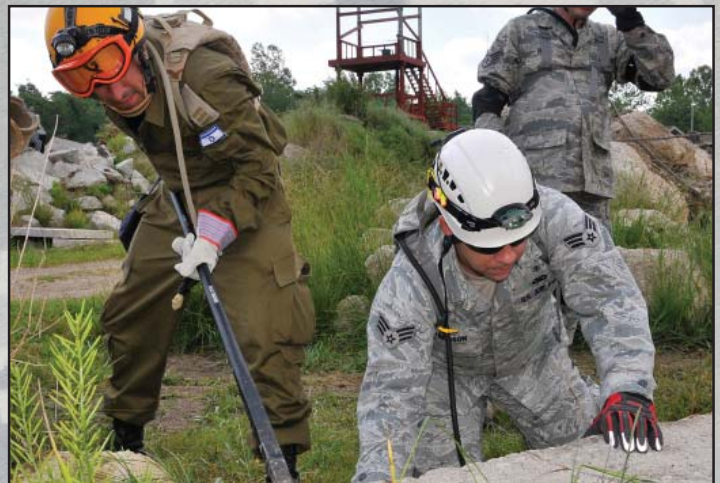
Air Force Senior Airman Micheal L. Atchison, 181st IW, 19th CERFP, along with an Israeli soldier, use a crowbar to lift and move heavy slabs of concrete at Camp Atterbury, Ind., June 10, 2013. (U.S. Air National Guard photo by Senior Master Sgt. John S. Chapman/Released)
