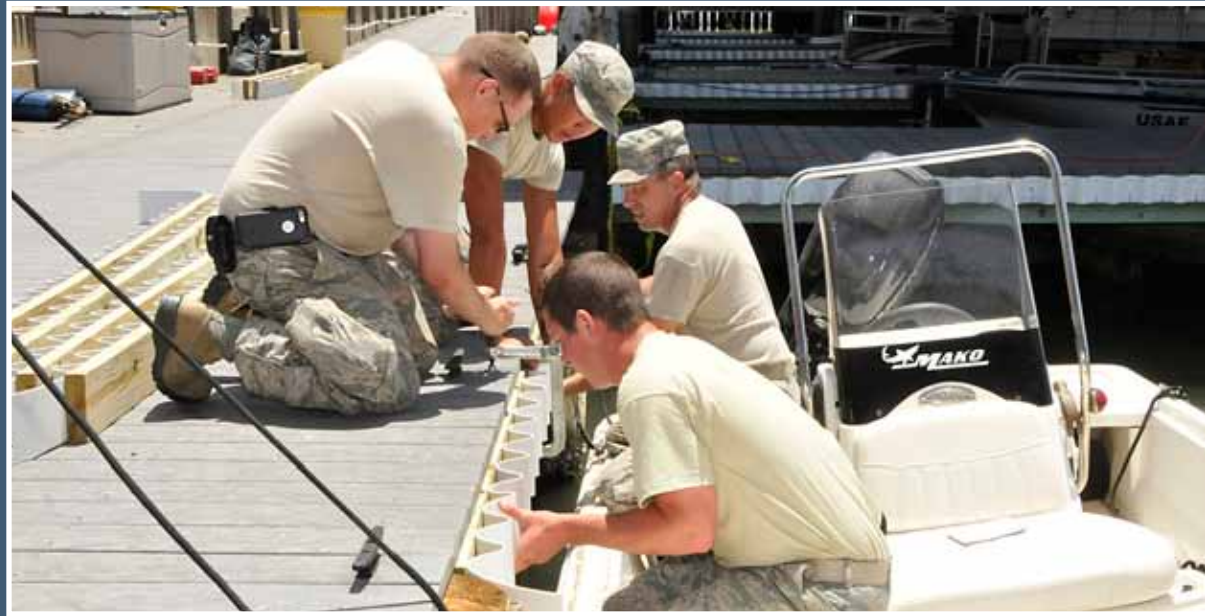
U.S. Airmen with the 181st Intelligence Wing Civil Engineering Squadron and 45th Space Wing Civil Engineering Squadron work together to install new dock fenders at the outdoor marina at Patrick Air Force Base, July 20, 2016. (U.S. Air National Guard photo by Senior Master Sgt. John S. Chapman)
