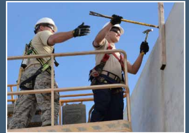
U.S. Airmen assigned to the 181st Intelligence Wing Civil Engineering Squadron, remove the safety line from the top of the building they are constructing during their annual training at Andersen AFB, Guam, July 14, 2016. The 181st engineers provided contingency related hands-on training for Air National Guard CE Airmen. (U.S. Air National Guard photo by Senior Airman Lonnie Wiram)
